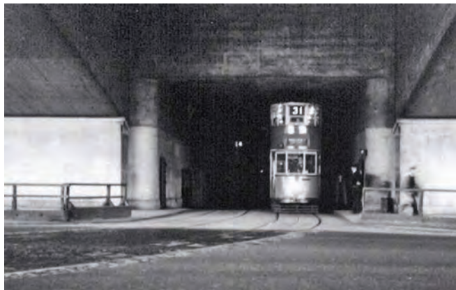
The south end of the Kingsway tram tunnel below Waterloo Bridge
